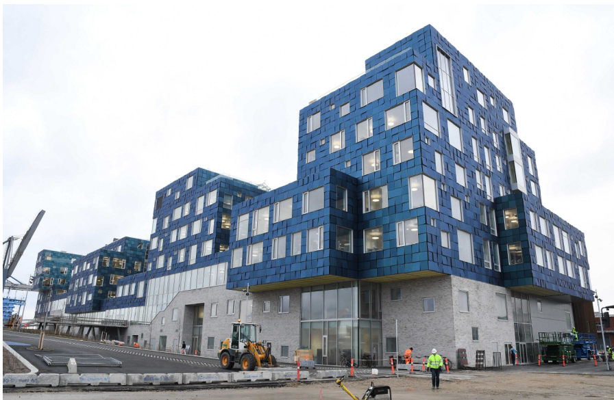
Figure 1: PV installation on Copenhagen International School inspired by this project.
