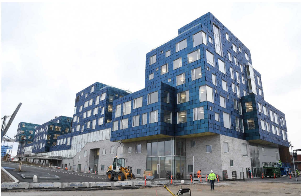
Figure 4: New Campus for Copenhagen International School the blue façade modules are solar panels with Swissinso glass.
